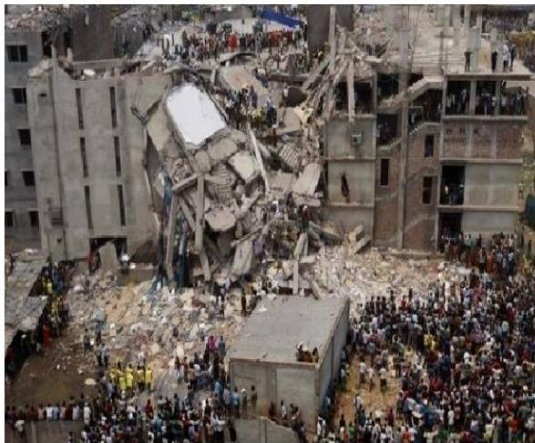
Figure 1: Collapse of Buildings
